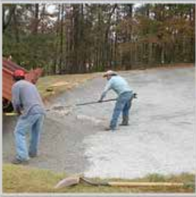
2. Install 2" layer of local gravel
