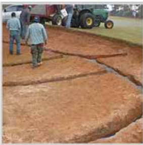
1. Remove old sand and inspect drain lines
