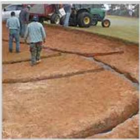
*1. Remove old sand and inspect drain lines*
